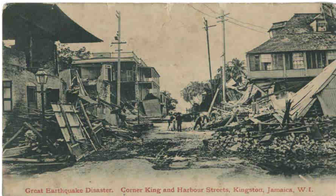
Great Earthquake Disaster, Corner King and Harbour Streets Image Courtesy of the National Library of Jamaica
