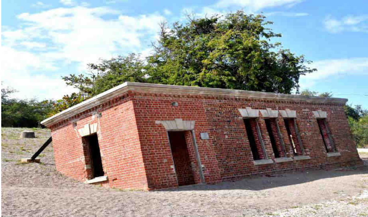
The Old Artillery Store in Port Royal (the Giddy House) tilted by the 1907 Earthquake Photo Courtesy of the JN Foundation
