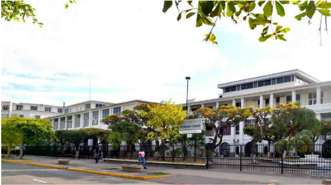
The Supreme Court Buildings on King Street Photo Courtesy of the JN Foundation
