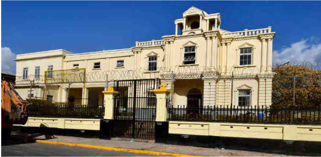
Kingston Technical High School Photo Courtesy of the JN Foundation
