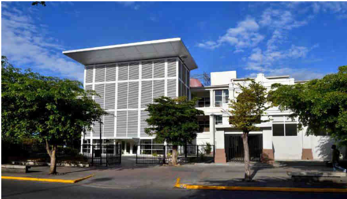
Court Buildings on King Street Photo Courtesy of the JN Foundation
