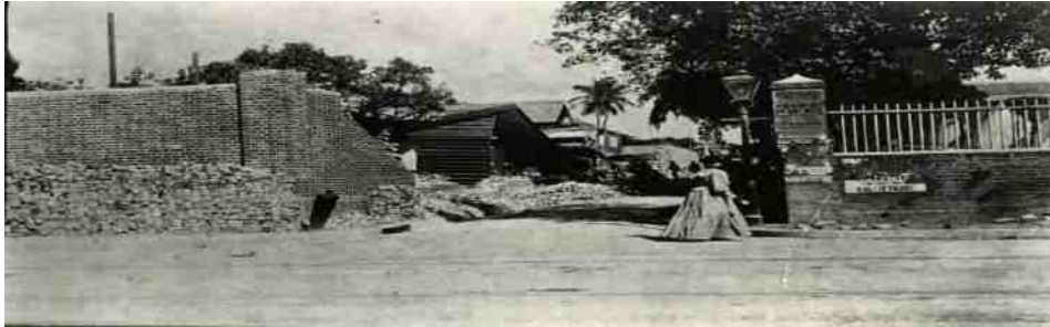
1907 Earthquake Destruction at the Old Wolmer's School Yard next to the Kingston Parish Church Image Courtesy of the National Library of Jamaica
