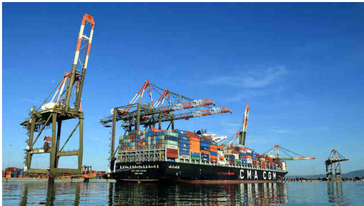
Container Ship Unloading at Kingston Wharves, Newport West Photo Courtesy of JN Foundation
