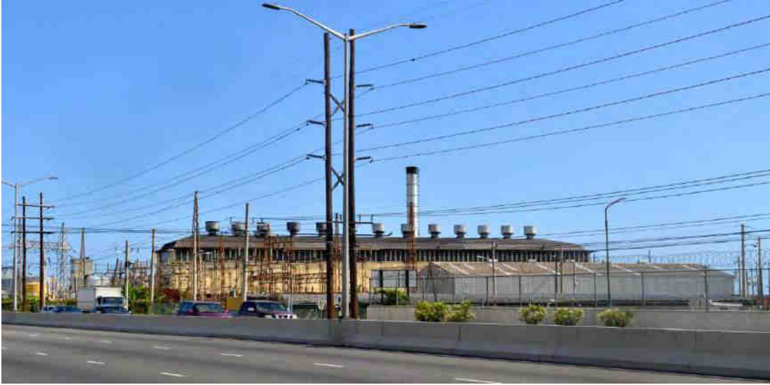
The Hunt's Bay Power Station on Lower Marcus Garvey Drive Photo Courtesy of the JN Foundation
