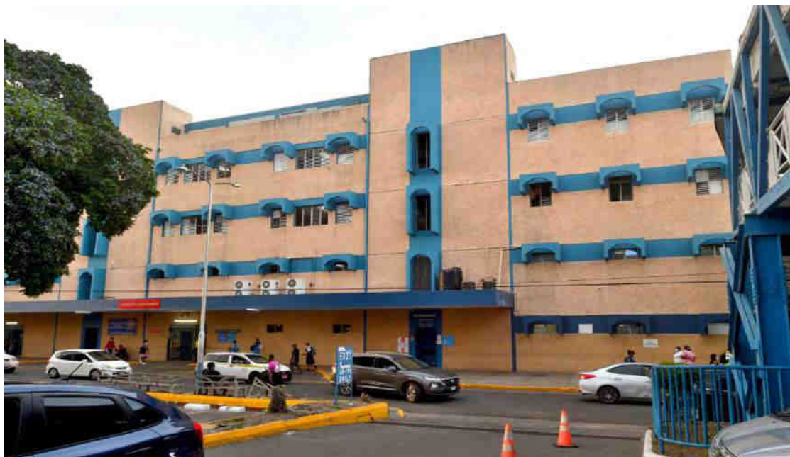
Entrance to the Kingston Public Hospital Photo Courtesy of the JN Foundation
