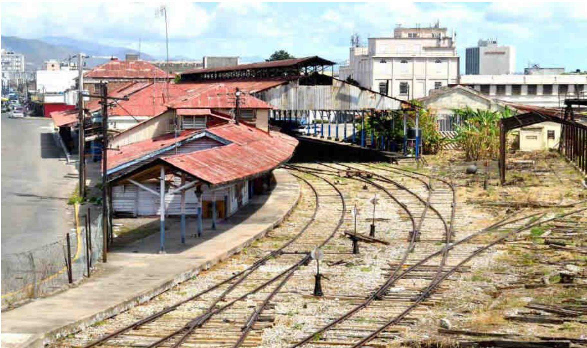
A View of the Jamaica Railway Station with Rail lines Photo Courtesy of the JN Foundation
