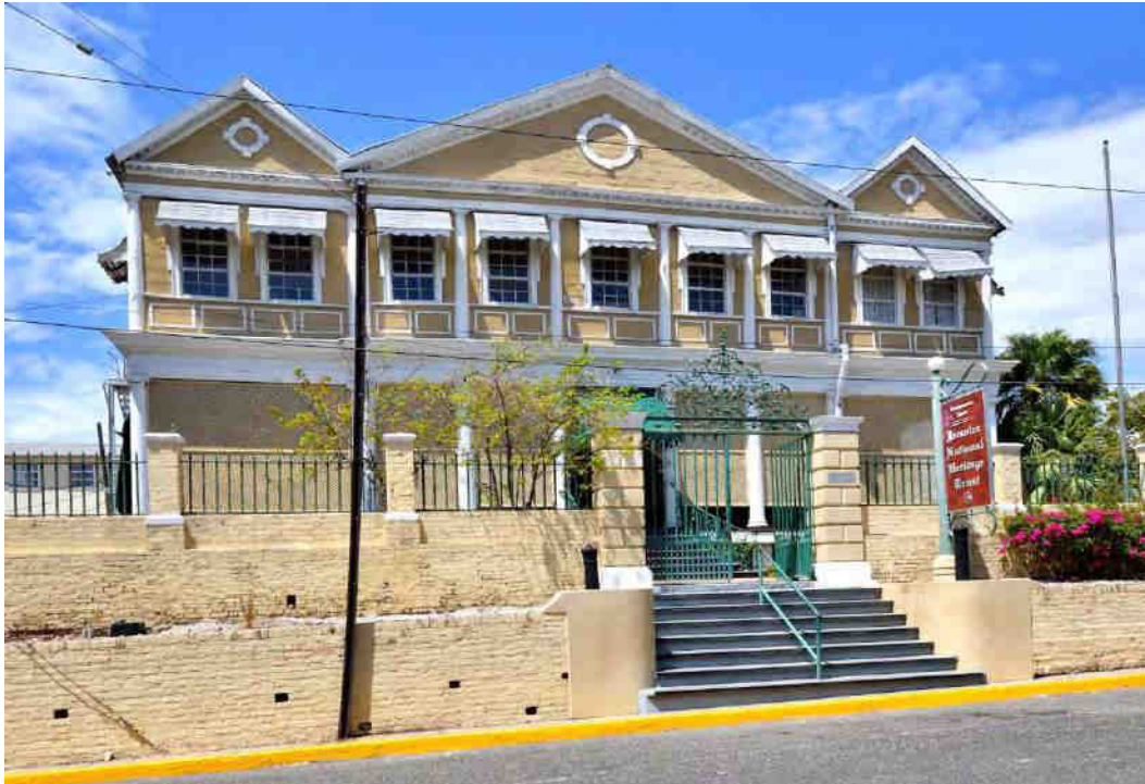
The Former Hibbert House/Headquarters' House, now home to the Jamaica National Heritage Trust Photo Courtesy of the JN Foundation
