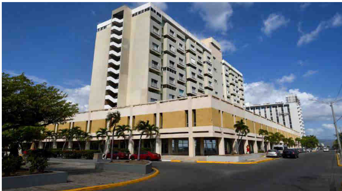
Views of Ocean Boulevard Photo Courtesy of the JN Foundation
