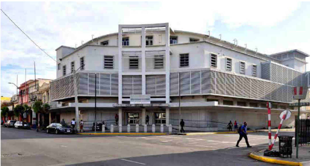
Part of the Supreme Court Buildings Photo Courtesy of the JN Foundation
